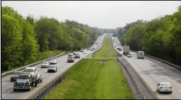
Figure 4. I-71 Northbound Approaching I-265
